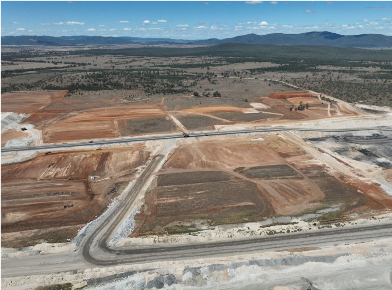
Figure 2: Image of recent clearing and soil stockpiles
